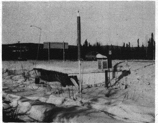
Figure 4. Farmer's Loop Road snow shed.
