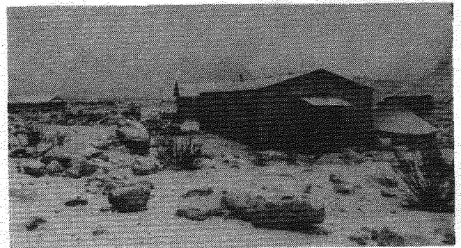
Fig. 8 Temporary Shelter of Corrugated Sheets
