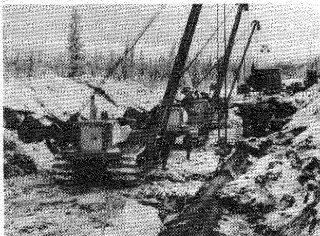
Fig. 5. Lifting the Operating Pipeline with Sidebooms at Milepost 720
