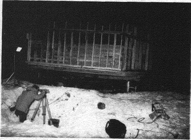
Fig. 1 Photo of pile loading system
