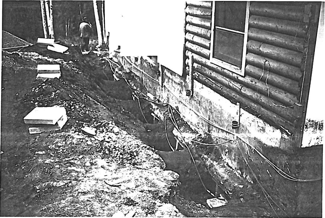
Figure 2c Pillow Jacks Installed Beneath the Footing
